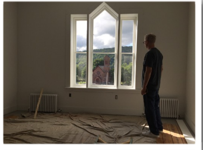
Partway through renovations, Gavin Maloney surveys the Little Falls skyline from the second floor of 600 Main Street.
